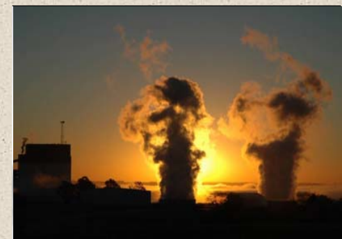
Co-firing switchgrass with coal..... the dawning of a new era.
