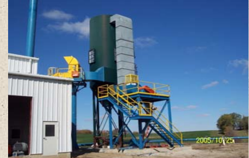
The ground switchgrass moves through the baghouse....
