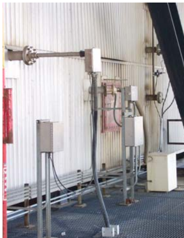
CEMS Probes In Outlet Duct
