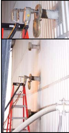
Emissions Probe In Outlet Duct
