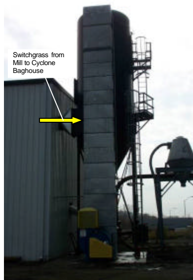
Cyclone Baghouse that conveys ground switchgrass from the "Eliminator" onto the Surge Bin Feed Conveyor and removes and filters dust from the processing area.
