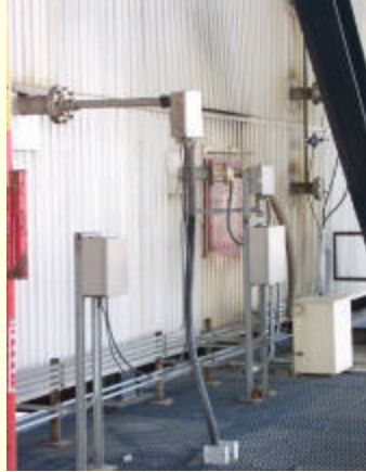
CEMS Probes In Outlet Duct
