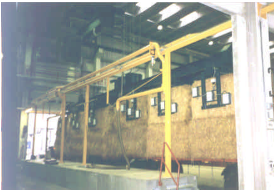
Figure 4.2 Unloading straw at Studstrup Power Station.
