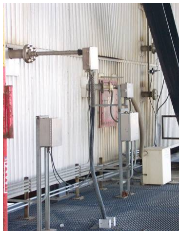
CEMS Probes In Outlet Duct
