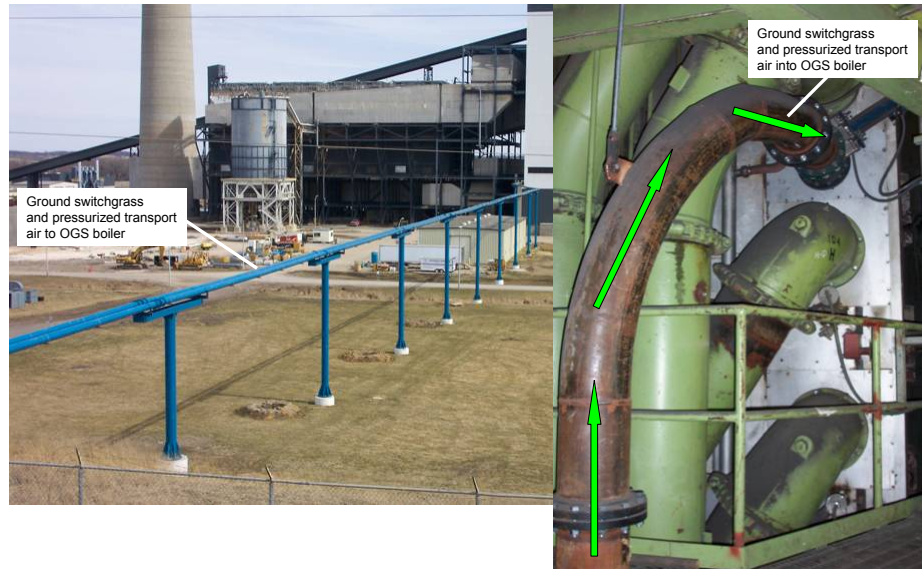
Switchgrass Blow Lines Transporting Ground Switchgrass into Boiler House (left) and Boiler (right).
