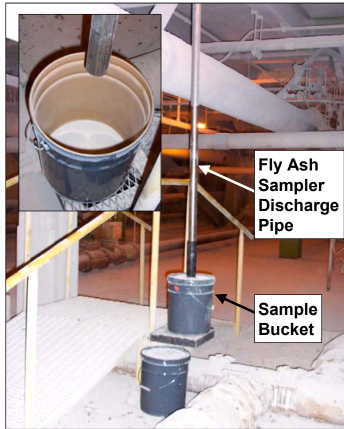
Exhibit 5: Discharge Pipe and Sample Collection Bucket for Automatic Fly Ash Sampler
