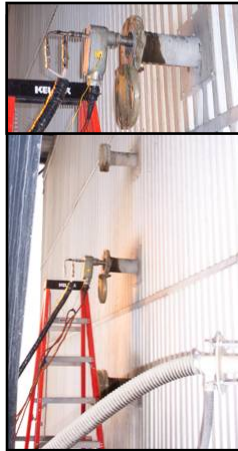
Emissions Probe In Outlet Duct
