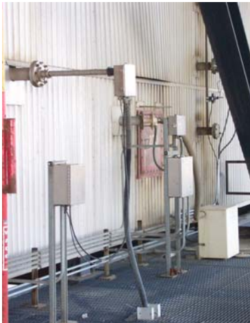
CEMS Probes In Outlet Duct
