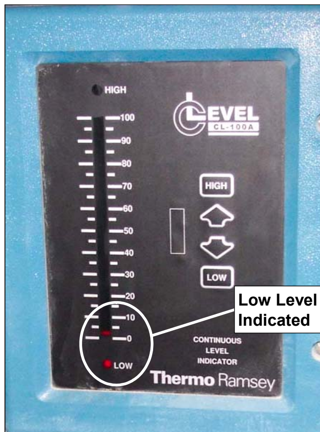
Exhibit 9: Low Level Indication on the Fly Ash Silo Level Indicator, Just Prior to Taking the Bulk Sample of Fly Ash from Cofire Testing on December 10, 2003.
