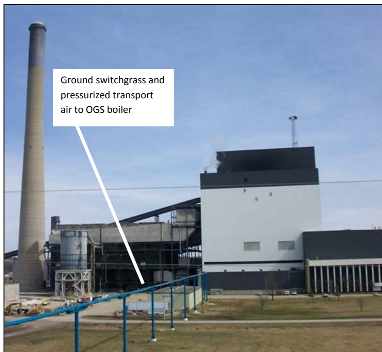
Exhibit 38 Processed Biomass Transport to Boiler
