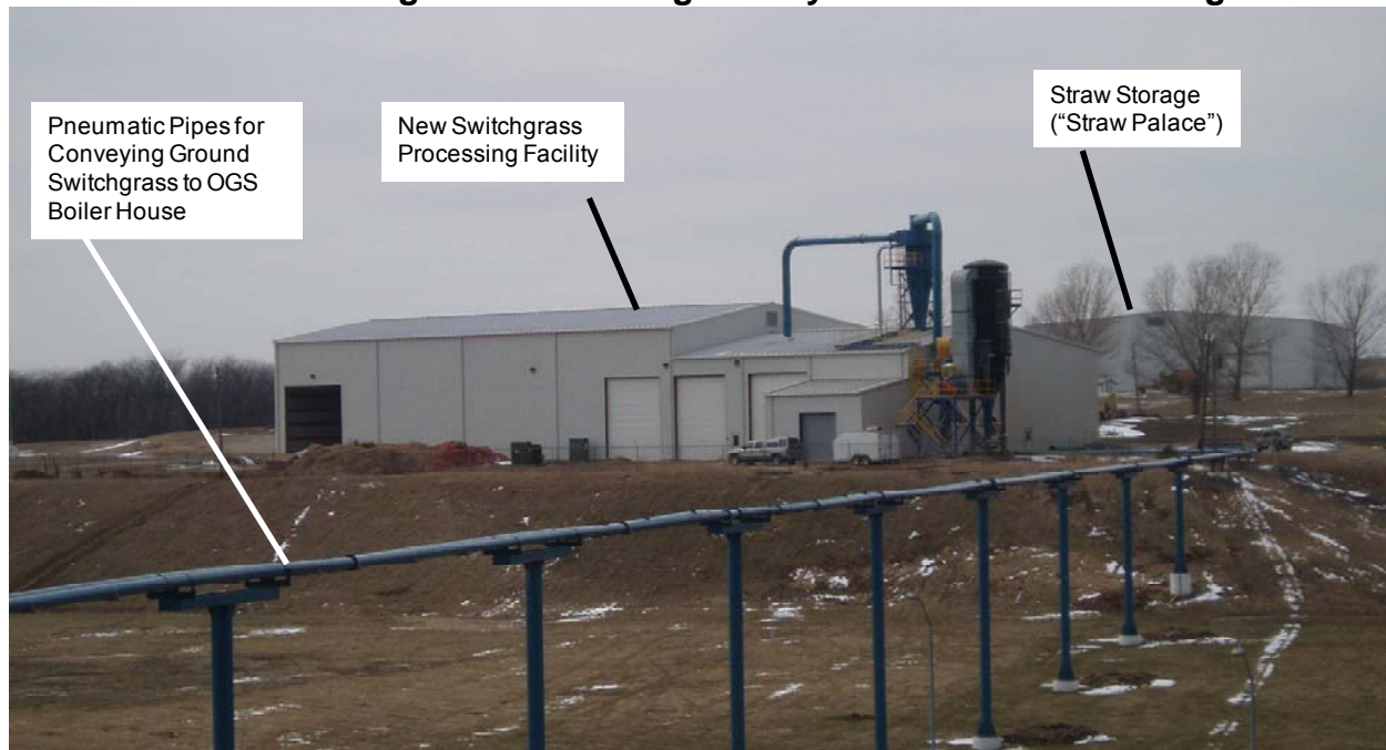
Exhibit 4 New Switchgrass Processing Facility at Ottumwa Generating Station
