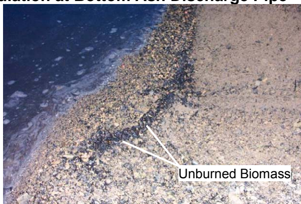
Unburned Biomass Accumulation
