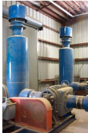
Exhibit 37 Photo of Pneumatic Blowers for Biomass Transport
