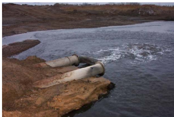
Bottom Ash Discharge Pipes
